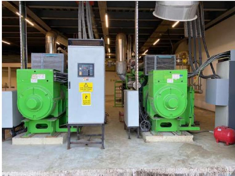
Electric generators from Biogas ( $3 \text{ Mwh}_{\text{elc.}}$ ) and heat ( $3 \text{ Mwh}_{\text{th}}$ ). This waste heat is used to dry the treatment sludge.
