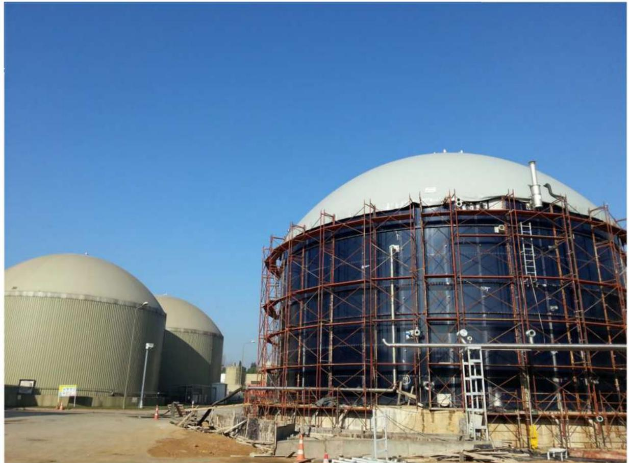
An anaerobic sludge digestion and thermal drying system is constructed for the wastewater treatment plant sludge. The biogas produced is used to generate electricity ( $3 \text{ Mwh}_{\text{elc.}}$ ) and heat ( $3 \text{ Mwh}_{\text{th}}$ ). This waste heat is used to dry the treatment sludge.
