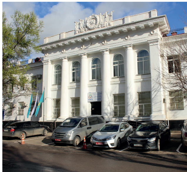
The CICA Secretariat's premises following relocation to Astana, 2016-2021
