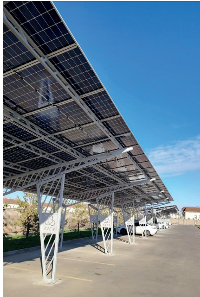
China: Solar power modules (DeepBlue, JA Solar company)
